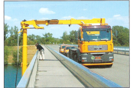
MBL 1600 T on Highway-Bridge Wien, Austria
